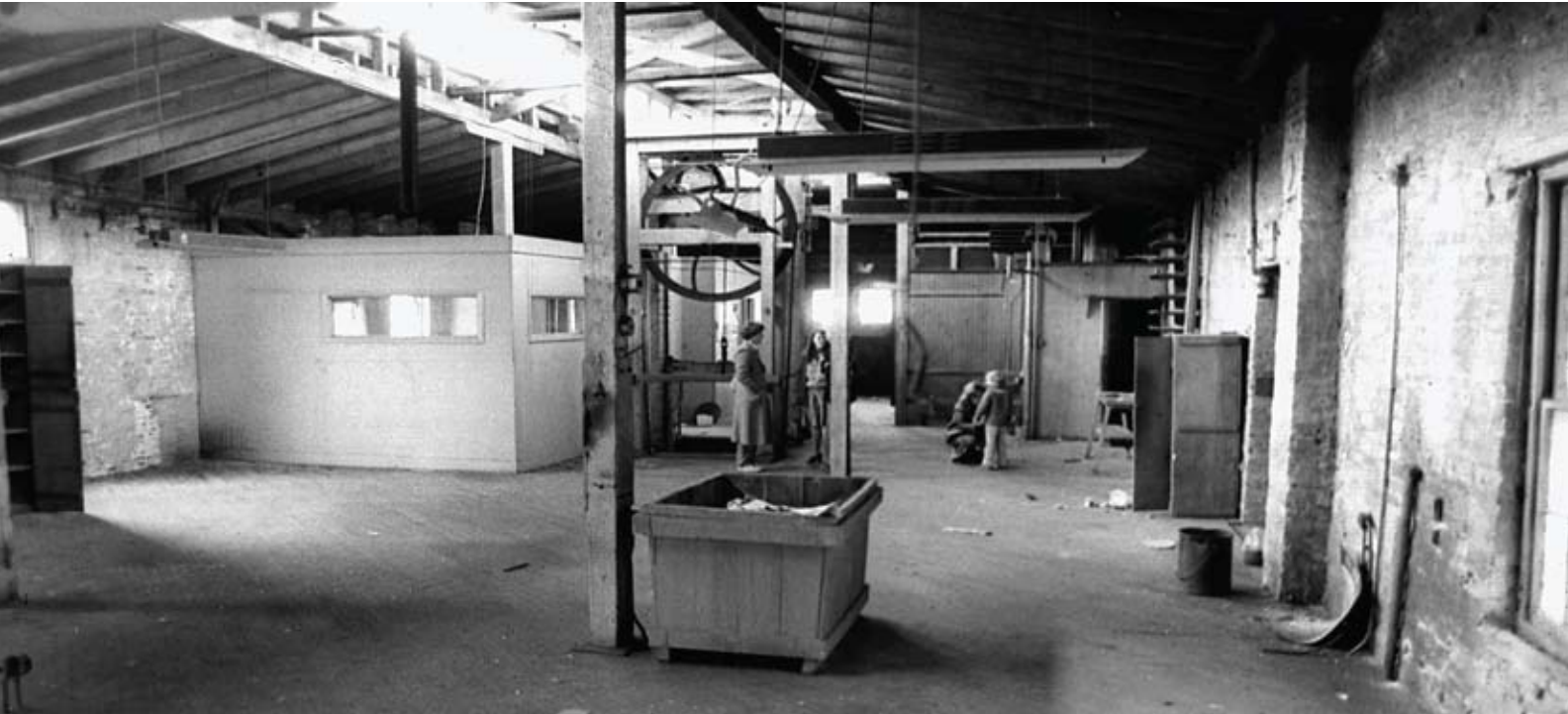
The second floor of the factory became DCCA's gallery.
